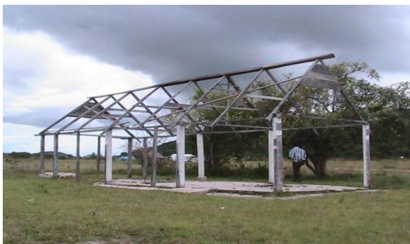
Dismantled village kitchen
